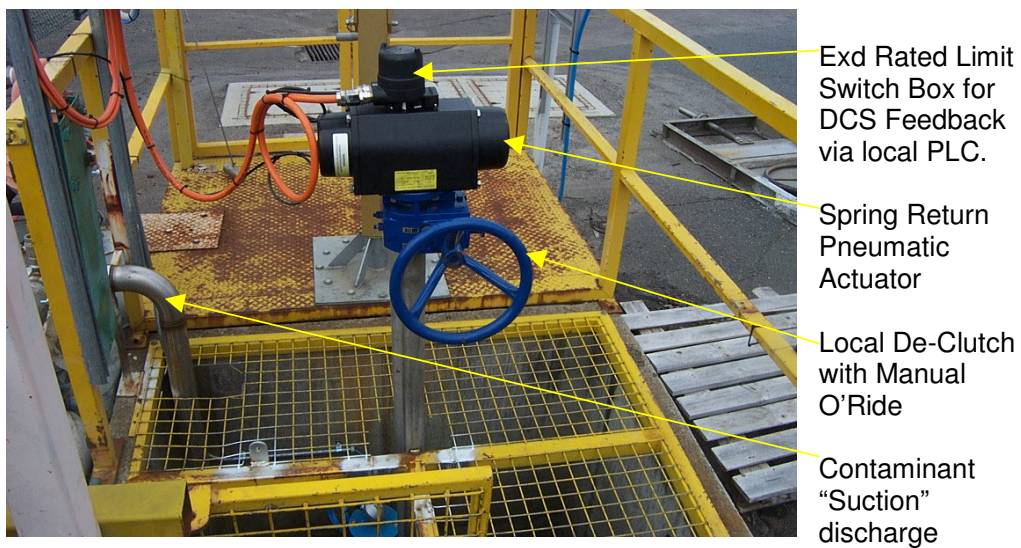
Figure 4.0 – Automatic control system with local manual override
